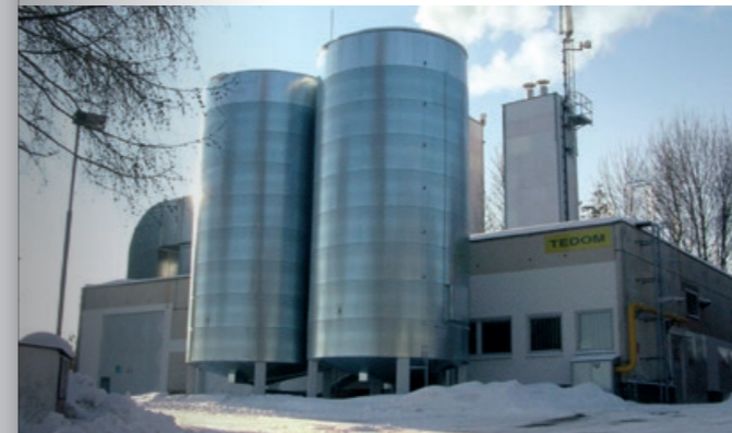
District Heating Plant, Světlá n. Sázavou, Czech Republic
